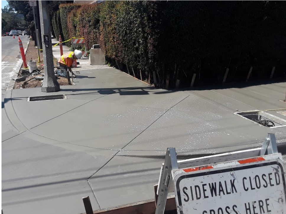
New access ramp at the corner of Mission and Bath Streets
