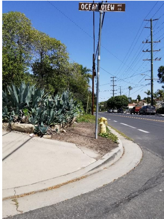
Missing sidewalk links on Old Coast Highway
