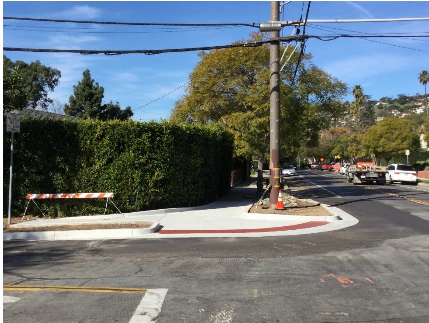
Completed sidewalk and curb ramp construction
